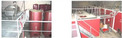
The catwalk around the pneumatic press.
